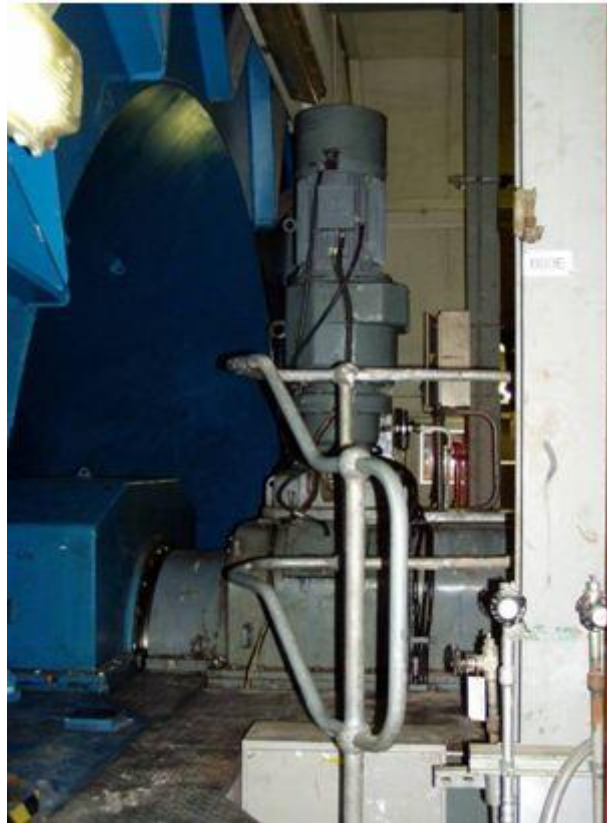
Figure 55 A barring motor in a power station alternator
